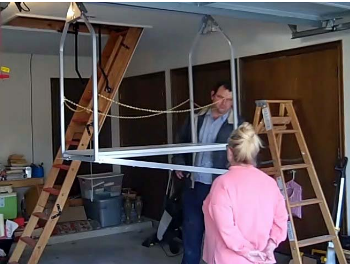
PHOTO SHOWING INSTALLER PULLING DOWN ON SPRING LOADED CEILING COVER.
